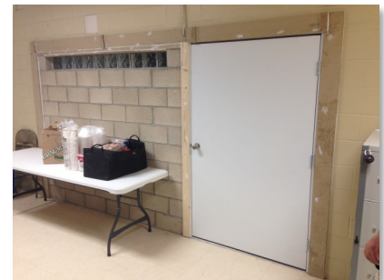
The New Club House Door
